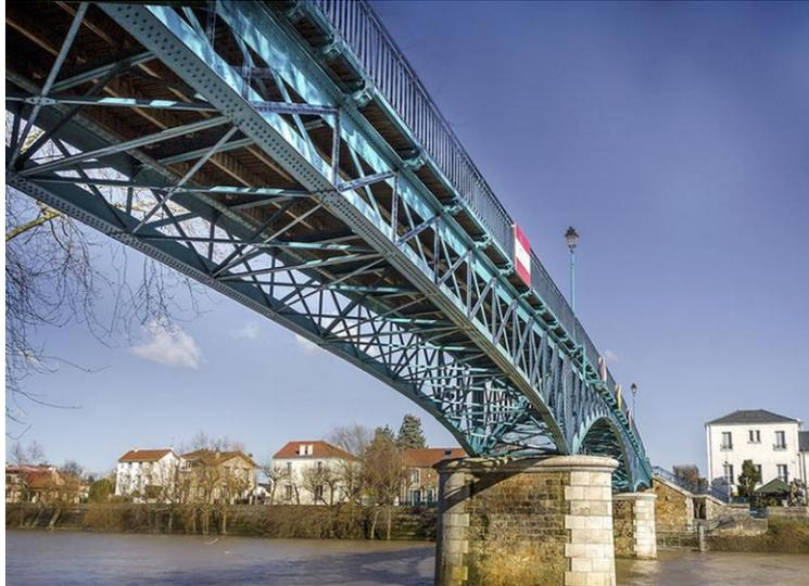
**Bry footbridge (above):** in order to make connections between the northern part of Bry and Le Perreux easier, a footbridge was built in 1893-94. Produced by the workshops of Gustave EIFFEL, it is an 80m-long metal structure resting on two river piers. The gangway was raised in 1917 to increase the draft. Reserved for pedestrians, it was transferred to the two towns of Bry and Perreux in 2007.
